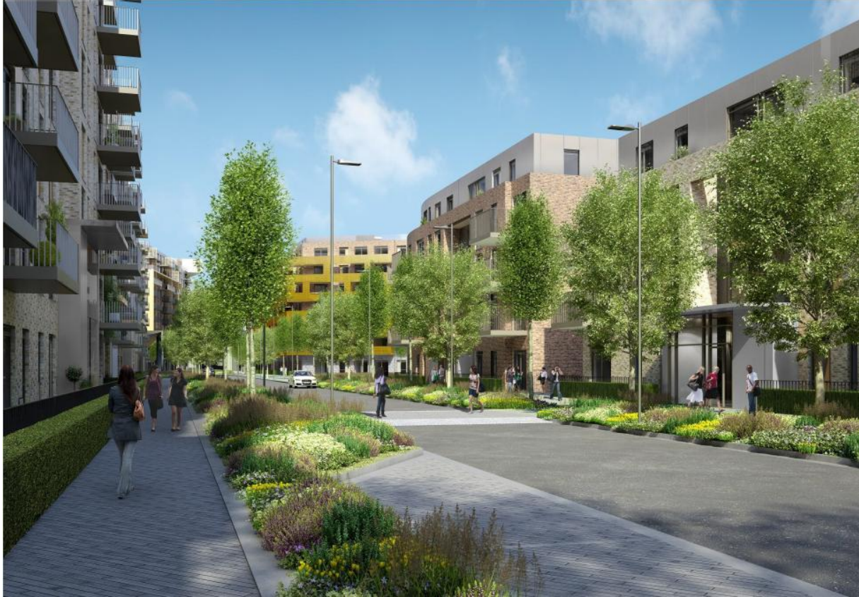
Looking North along Mary Neuner Road
